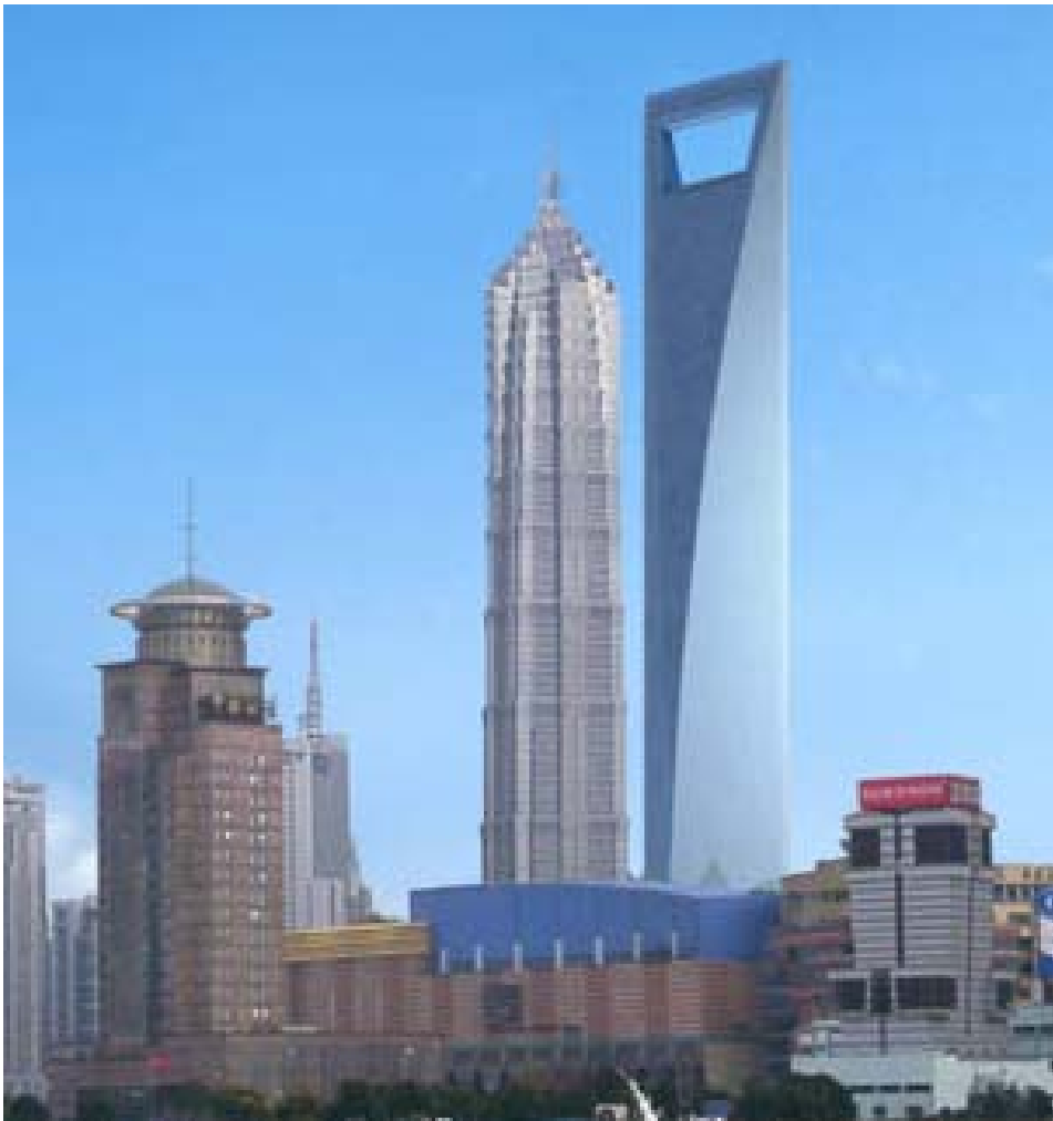
WFC, Shanghai Grade 450 steel, 100mm thick
