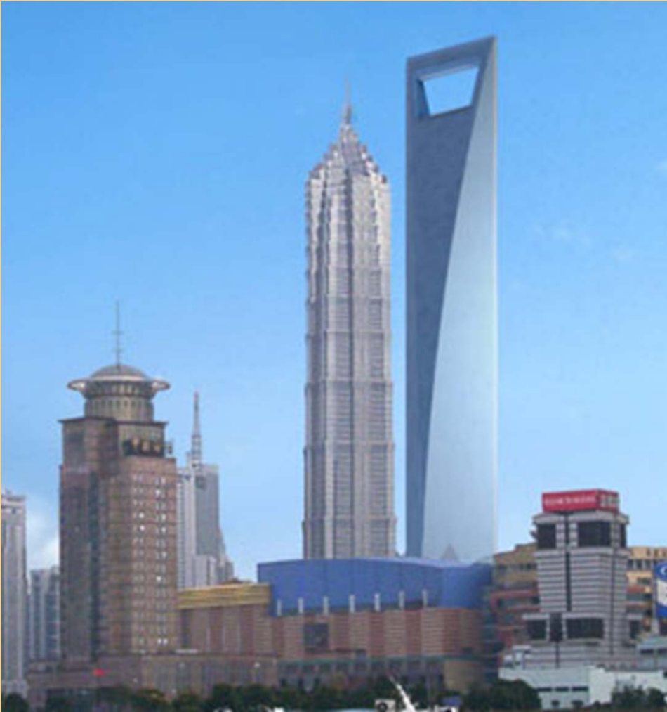
WFC, Shanghai Grade 450 steel, 100mm thick
