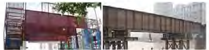
Figure 3: Plate girder
